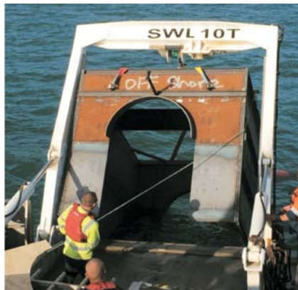
The NZ Diving & Salvage Ltd crew in the process of lowering the metal box, part of the manufactured repair solution, to the outfall pipe. The box weighs over a tonne.
