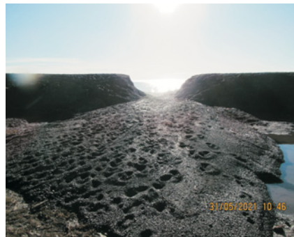
Figure 1: Breach of the sacrificial gravel embankment at Westshore caused by the swell event in May 2021.
