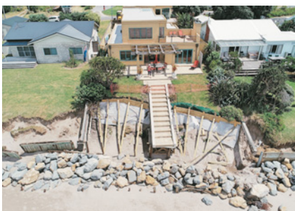
Figure 3: Drone footage of the eroded area showing the remains of the old retaining wall, and the temporary rock revetment. Geotextile was placed along the top of the bank in an attempt to protect it from further erosion.
