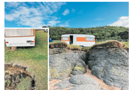
Figure 5: Caravan set up at the summer camping area at Turihaua Point showing the channels formed in the low cliff that direct water towards the campers during high sea events. (Inset) Channel cut in the sea cliff immediately behind the caravan showing recent collapse of top soil and the discolouration from salt burn of the grass.
