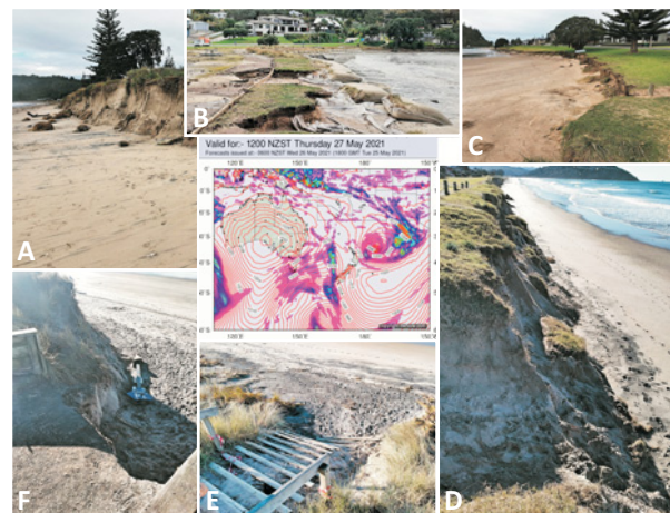
Figure 1: Impacts of the swell event on east coast shorelines. (A) Shoreline erosion at southern Whangamata Beach (Pipi Rd reserve area); (B) Brophy's Beach geotextile wall; (C) Whangamata harbour reserve erosion; (D) southern Pauanui Beach; (E) and (F) damaged beach accessways Whangamata.
