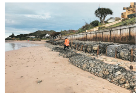
Figure 2: South Wainui Beach, Gisborne showing the old retaining wall and damaged gabions prior to the storm surge.
