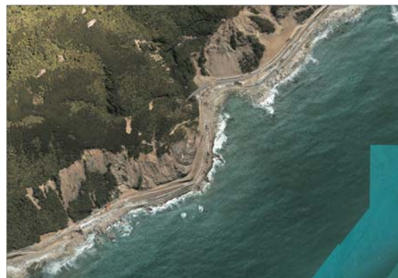
SH1 at Ōhau Point in December 2016 (top) and in November 2017 (bottom) (Photos: NCTIR).
