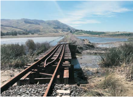
Rail Bridge 129 at Tirohanga post-quake (Photo: NTCIR).
