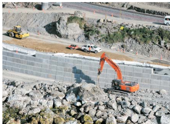
Seawall construction work underway near Ōhau Point (Photo: NTCIR).
