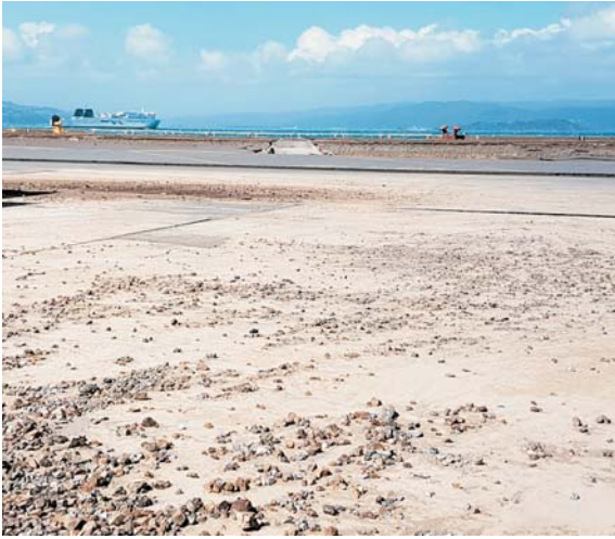
Liquefaction within the container terminal (Photo: CentrePort).
