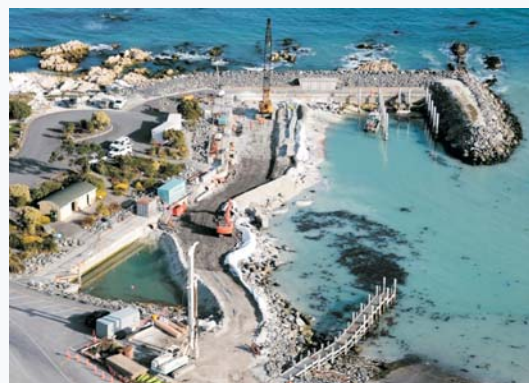
Work underway on repairing Kaikōura Harbour (Photo: NTCIR).
