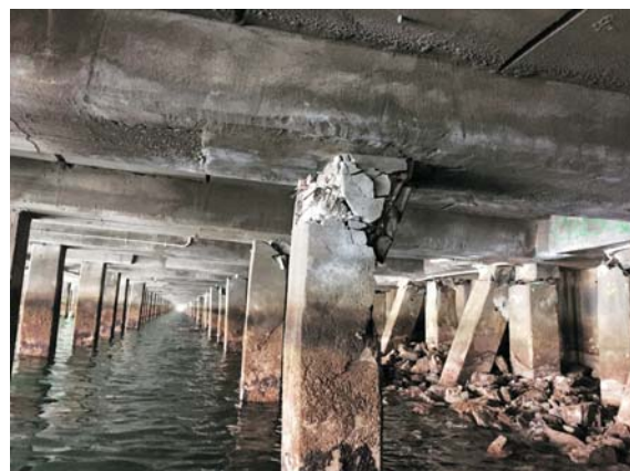
Pile damage under Thorndon Container Wharf (Photo: CentrePort).
