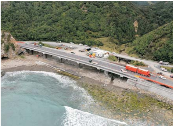
Work on the new, seven-span Irongate Bridge, north of Mangamaunu, nearing completion (Photo: NTCIR).
