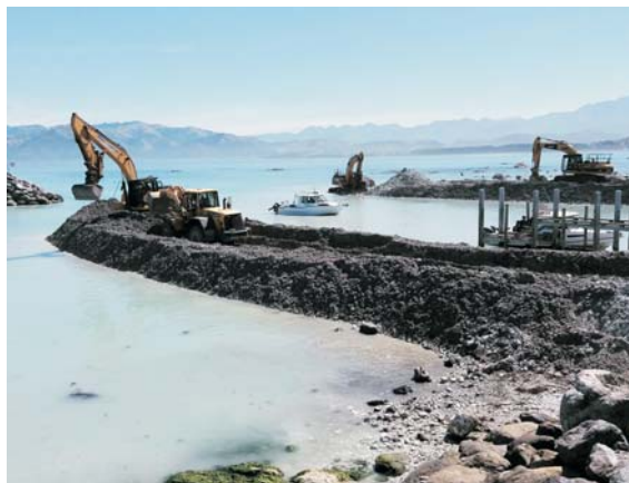
Kaikoura marina being dredged out to make it usable again (Photo: Hamish Rennie).
