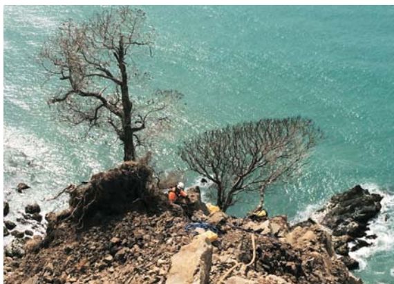
Abseilers clearing loose rocks to stabilise the cliff face (Photo: NTCIR).
