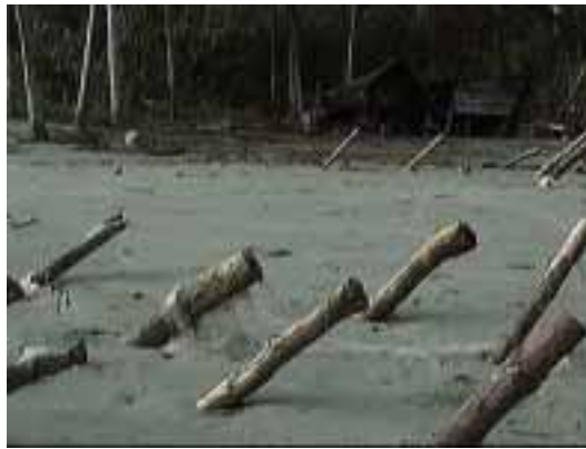
Remains of a house at Bliiri River. Houses in the foreground were totally destroyed, while those in the background were badly damaged. Wave height varied from 3 m to 11 m over a distance of about 250 m
