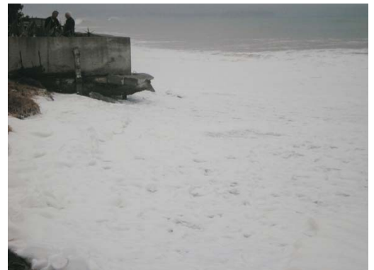
Wave action around a seawall on Clifton Road, Haumoana. Courtesy Hawke's Bay Regional Council.
