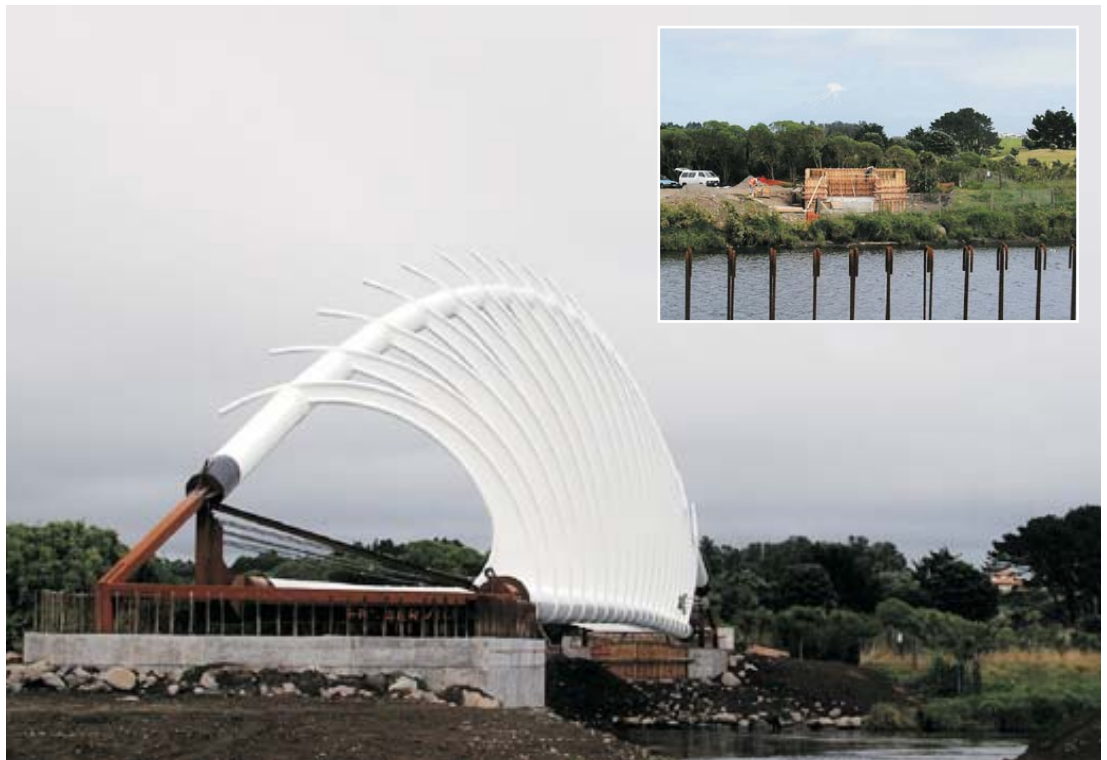
The bridge in place over the Waiwhakaiho River. Inset: Boxing for reinforced concrete and view across Waiwhakaiho River where Te Rewarewa Bridge will connect the existing and new section of the walkway. Both photos courtesy Whitaker Civil Engineering Ltd.
