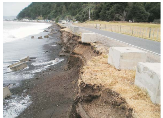
Erosion adjacent to the access road into Clifton Motor Camp. Courtesy Hawke's Bay Regional Council.
