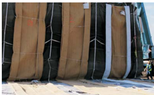
Figure 1: Geotextile bag construction for a multi-purpose reef. Courtesy ASR Ltd.
