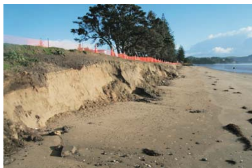
Figure 5: Orewa Beach erosion. Courtesy OBRCT.
