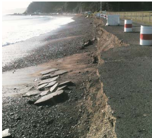
The access road to Clifton Motor Camp continues to be eroded as illustrated in the above photos. Photos: HBRC.
