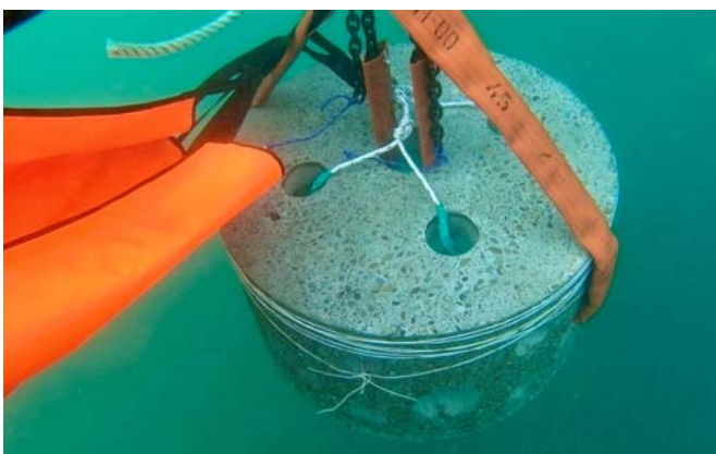
Figure 1: Deploying a Sea Nest in Bluff Harbour (Photo: Waka Miller, Sea Nest Ltd).
