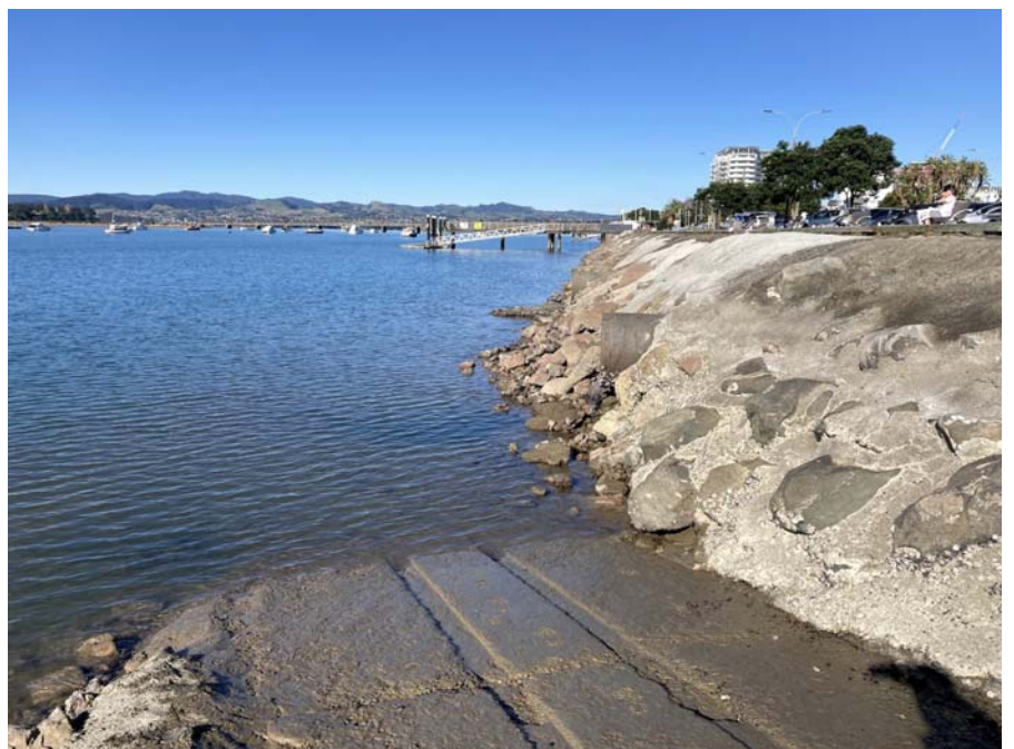
Figure 1: Existing seawall structure, June 2023 (Photo: WSP).
