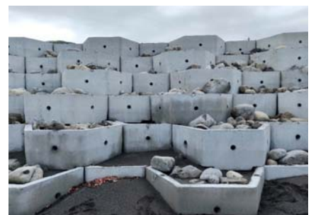
EcoReef cellular retaining walls.
