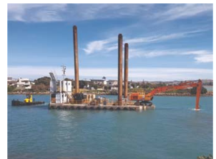
Figure 4: Dredge in operation at the Napier inner port entrance (Napier City Council).
