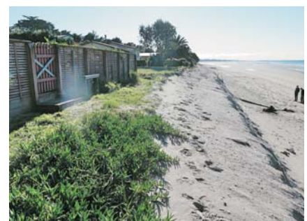
View north of 1126 Collingwood-Puponga Main Road beachfront 28 June 2019 (Photo: Eric Verstappen, Tasman District Council).
