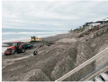
Pukehina Beach soft engineering (Photo: Paul Greenshields, BOPRC).
