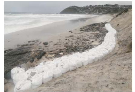
Temporary sand bag barrier on Middle Beach (Photo: Tom Simons-Smith, DCC).
