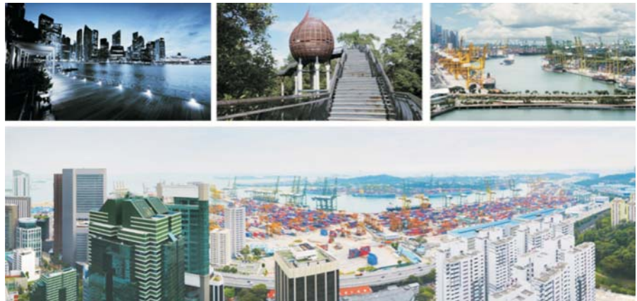
Figure 1: Singapore's varied coastline, clockwise from top left: Marina Bay; the Pungol Reserve; the causeway to Sentosa recreational island; and overlooking Keppel Port, which will be transferred to the west of the island by 2030 to create more space for commerce, residential developments and recreation (Photo source: Deposit Photos).
