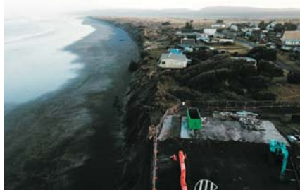
Sunset Beach (Port Waikato) coastal erosion (Photos: Waikato District Council).
