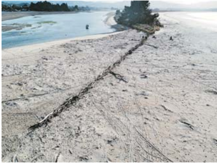
Aerial view of the driftwood windbreak on the day of construction. Fence alignment was determined based on the local wind conditions and took into consideration the way that the sand spit has accreted in the past (Photo: Tom Simons-Smith).
