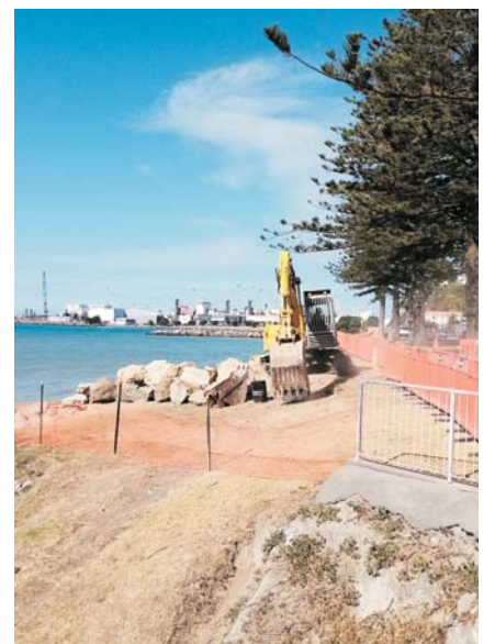
Figure 8: Hardinge Road coastal protection works, February 2020 (Photo: José Beyá).
