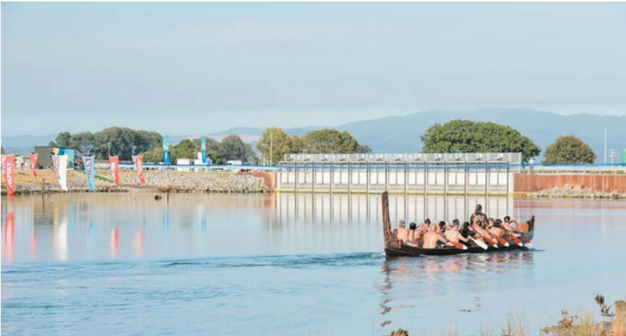
The Te Arawa waka paddling towards the Ford Road bridge’s 12 newly installed culverts (Photo: BOPRC).
