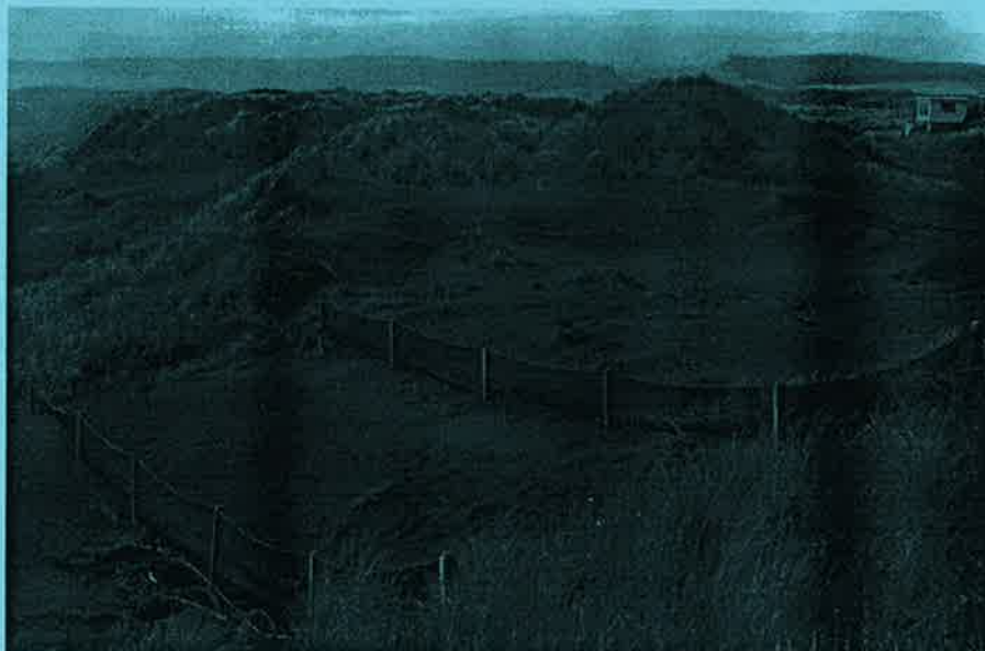
Wind erosion damage repaired using machinery and sand-trapping fences placed to hold the repaired dune in profile.
