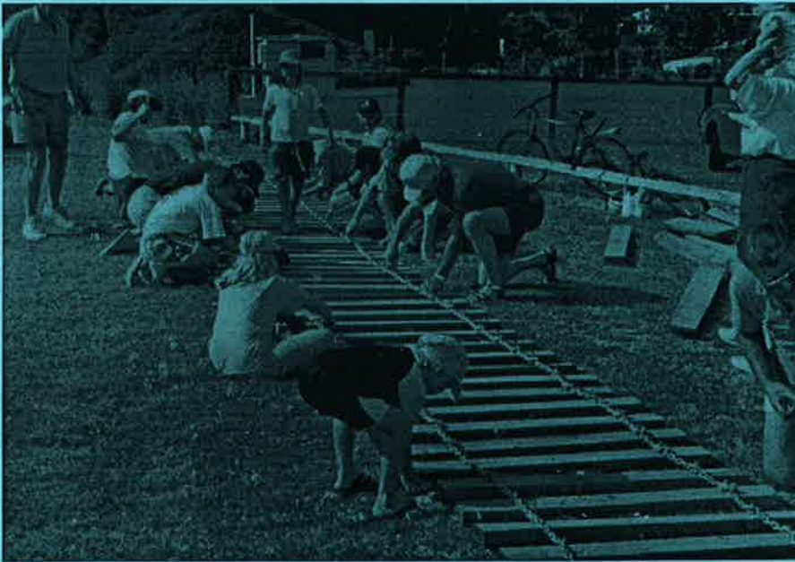
Beach Care members assembling a board and chain accessway for placement on Whiritoa Beach.
