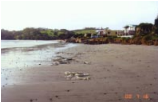
Figure 4: Cooks Beach showing the erosion of the dune toe exposing the rock works along the front of the beach. In the foreground are the tops of sand bags placed on the beach in 1978
