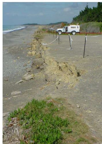
Figure 2: The Amberley Beach carpark after 3m of erosion following a storm in February 2002.
