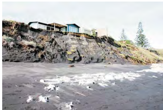
Erosion at Mokau. Photo courtesy of Environment Waikato.
