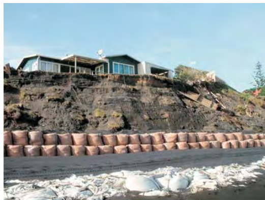
Temporary seawall at Mokau. Photo courtesy of Environment Waikato.
