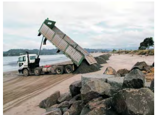
Sand replenishment at Buffalo Beach, Whitianga. Photo courtesy of Environment Waikato.
