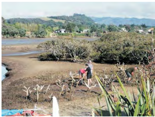
Mangrove Management work being done in Mangawhai Harbour. The Mangrove Management Support Programme is helping to fund this work. Credit: Ricky Eyre, Coastal Monitoring Officer at Northland Regional Council.
