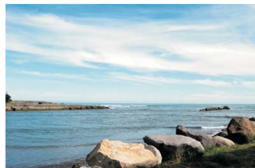
Waitara River mouth showing concrete training groynes and channel. Credit: Erin Zydervelt.
