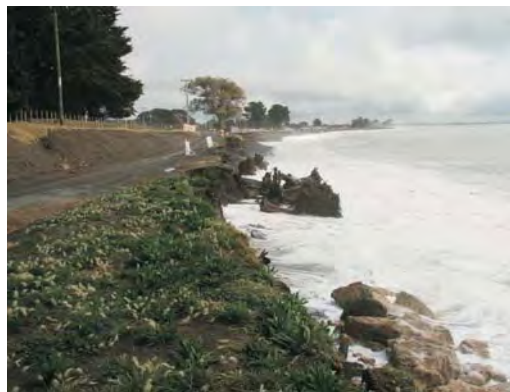
Vehicle access has been suspended due to safety concerns. Photo: HBRC.
