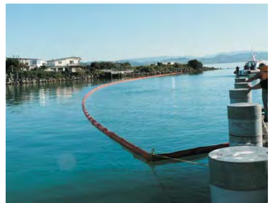
Rapid deployment boom in place, closing off the whole of the inner harbour. Photo: Neil Daykin, HBRC.
