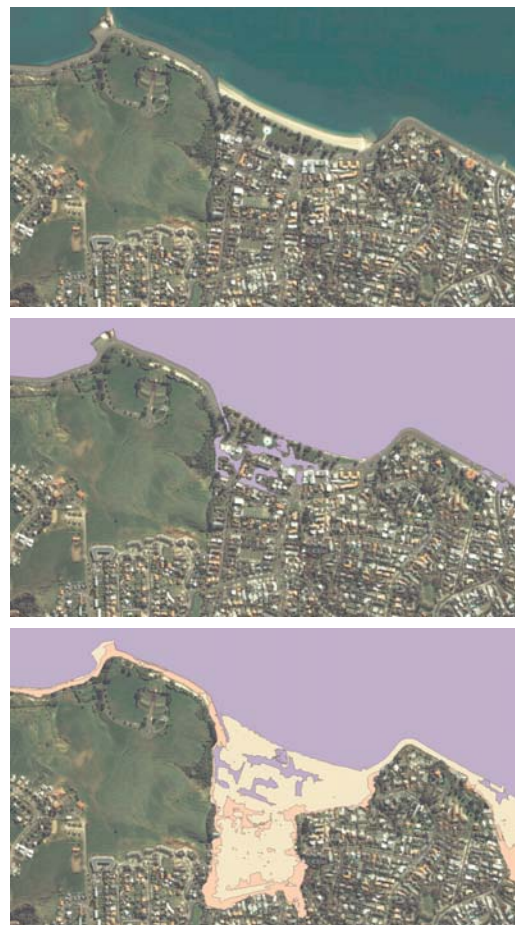
Top: Aerial photograph of Mission Bay. Centre: Mission Bay with present-day 1 per cent annual exceedance probability storm-tide plus wave set-up elevation superimposed (purple shading); Bottom: Mission Bay with present-day 1 per cent annual exceedance probability storm-tide plus wave set-up elevation superimposed (purple shading), plus 1-metre sea-level rise (light shading), and plus 2-metre sea-level rise (orange shading). Credit: NIWA.
