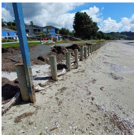
Snells Beach, Rodney: Failed timber seawall post event (Photos: Auckland Council).
