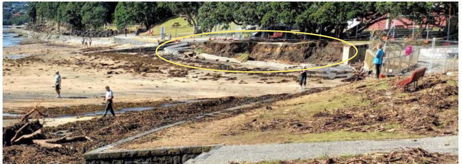
Murrays Bay, East Coast Bays: Failed section of seawall during and post the Cyclone Gabrielle storm (Photos: Auckland Council).
