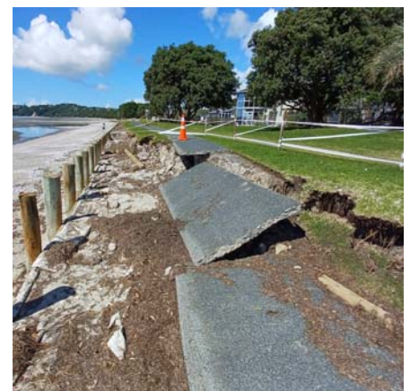
Snells Beach, Rodney: Failed timber seawall post event (Photos: Auckland Council).
