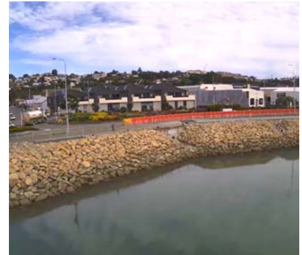
Site after Jull Wharf removal (Photo: NCC).
