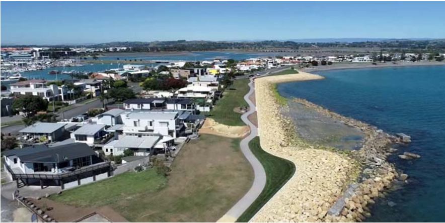
The completed Rangatira revetment (Photo: Napier City Council).
