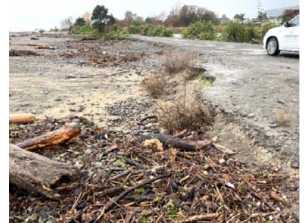
▲ Te Awanga: erosion of the Maraetotara River stopbank (top) and debris (bottom) (Photos: João Allbuquerque).
